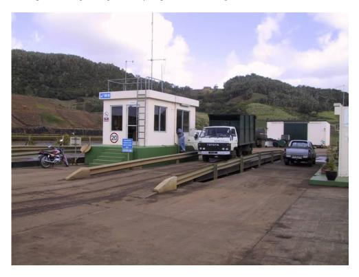
Figure 31 Electronic weighbridge for trucks delivering waste to the landfill
