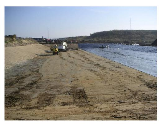
Figure 28 Construction of clay liner and installation of HDPE-liner
