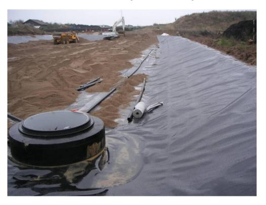
Figure 29 Installation of drainage layer on top of the HDPE-liner
